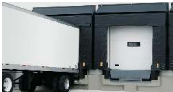
Figure 2 Example of "Dock-in" Shipping and Receiving doors
