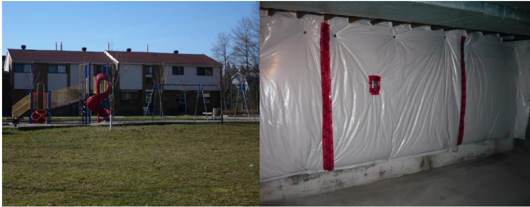
Figure 5.2, Cornwall Social Housing Exterior and interior view of installed basement insulation blanket
