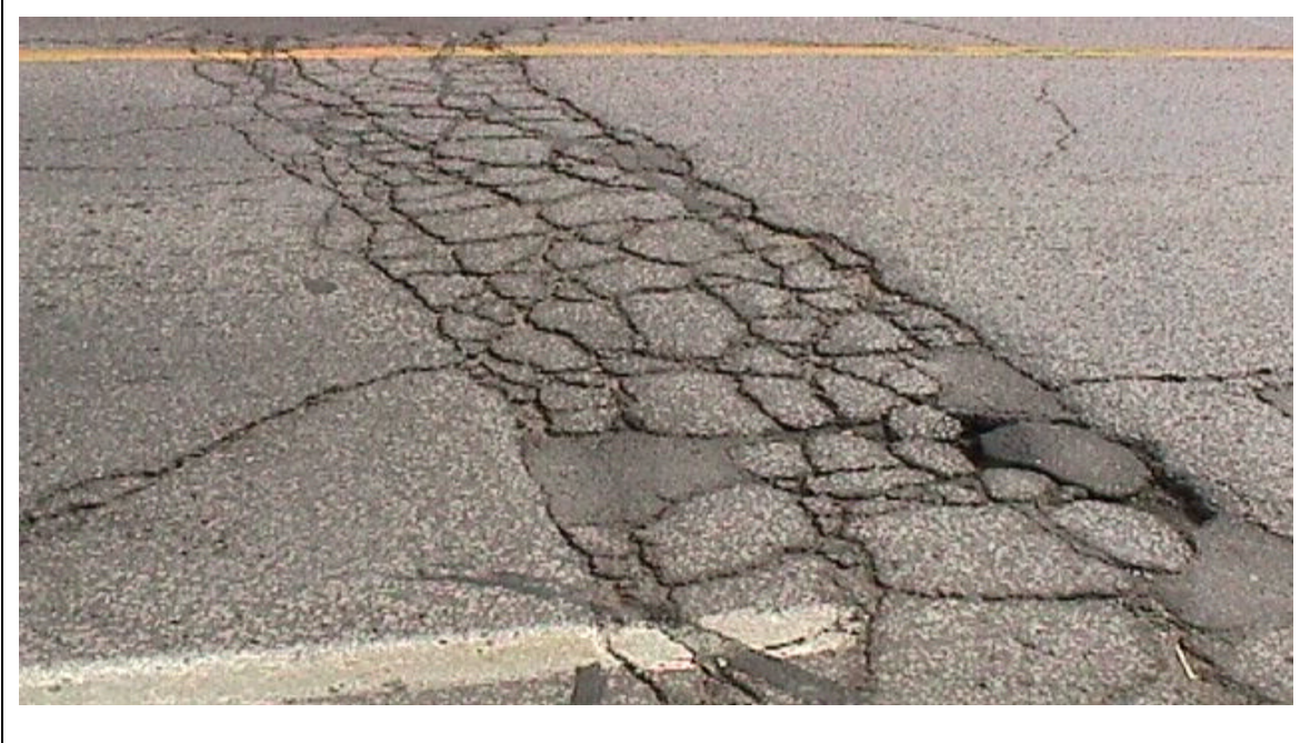
Figure 2 - Utility trenching damage to a pavement in Ottawa-Carleton
