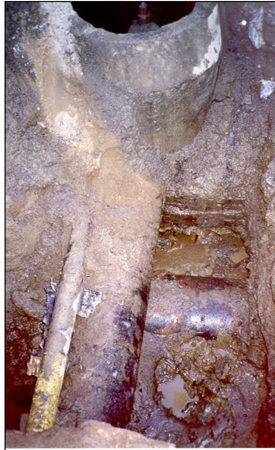
Figure 4 - Gas line (yellow, smaller pipe on top of the larger pipe ) situated on top of water main in Ottawa-Carleton
