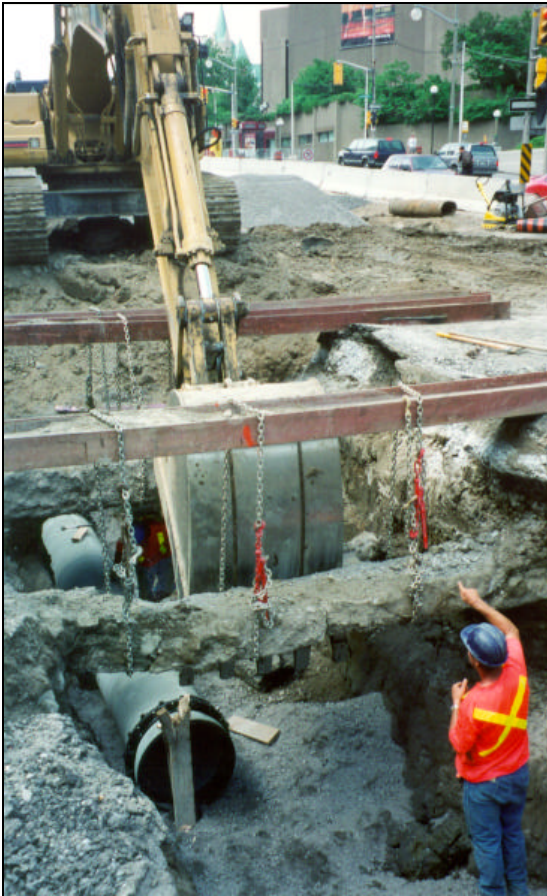
Figure 3 - Slowly working around shallow utility plant on Elgin Street in Ottawa-Carleton
