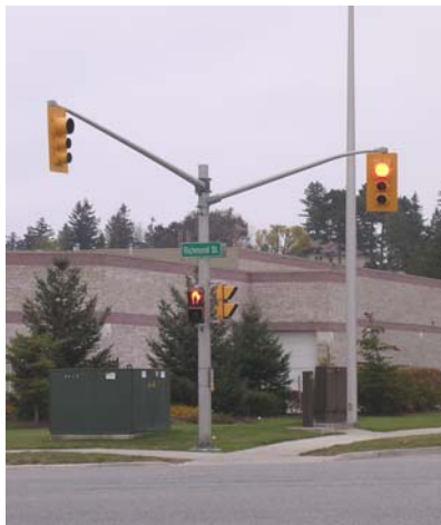
Figure 3-1, Signals Installed on One Corner of Typical Intersection
