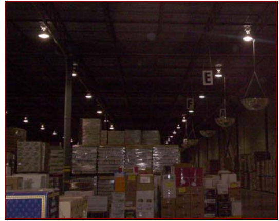
Figure 10-7, Metal-Halide Lighting in Expanded Warehouse
