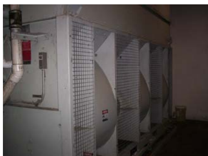
Figure 14-4, Cooling Tower Blowers
