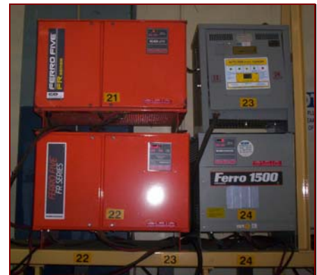
Figure 10-14, Typical Battery Chargers
