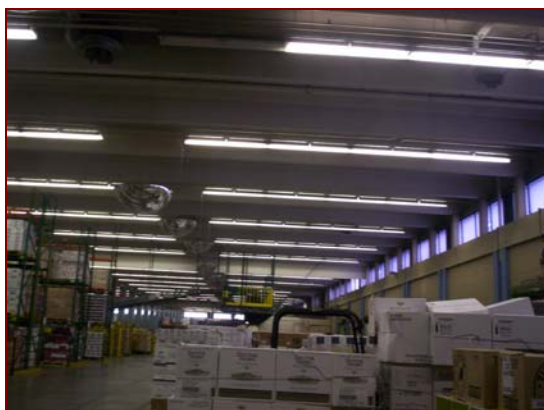
Figure 10-5, Suspended Fluorescent Fixtures in Original Warehouse
