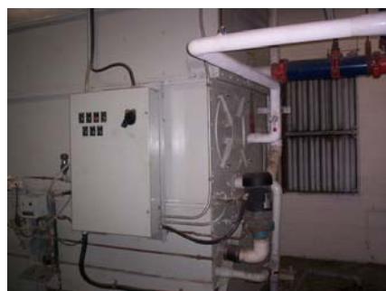
Figure 14-4, Cooling Tower Blowers
