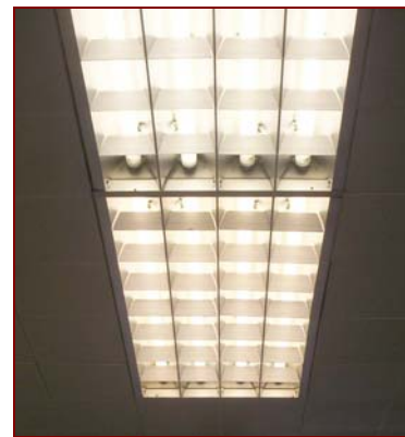
Figure 10-12, Existing 4-Lamp Fixtures in Office Area
