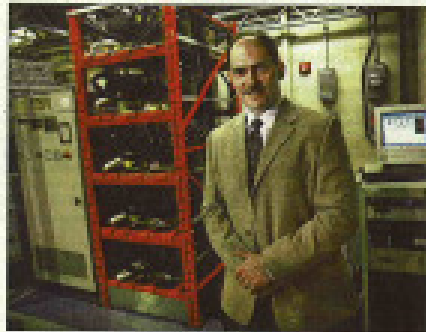
Halton Hills Hydro president Dan Guatto says the firm's power project uses Swiss-made batteries to store electricity at night when demand is lower, with power discharged during peak periods.
