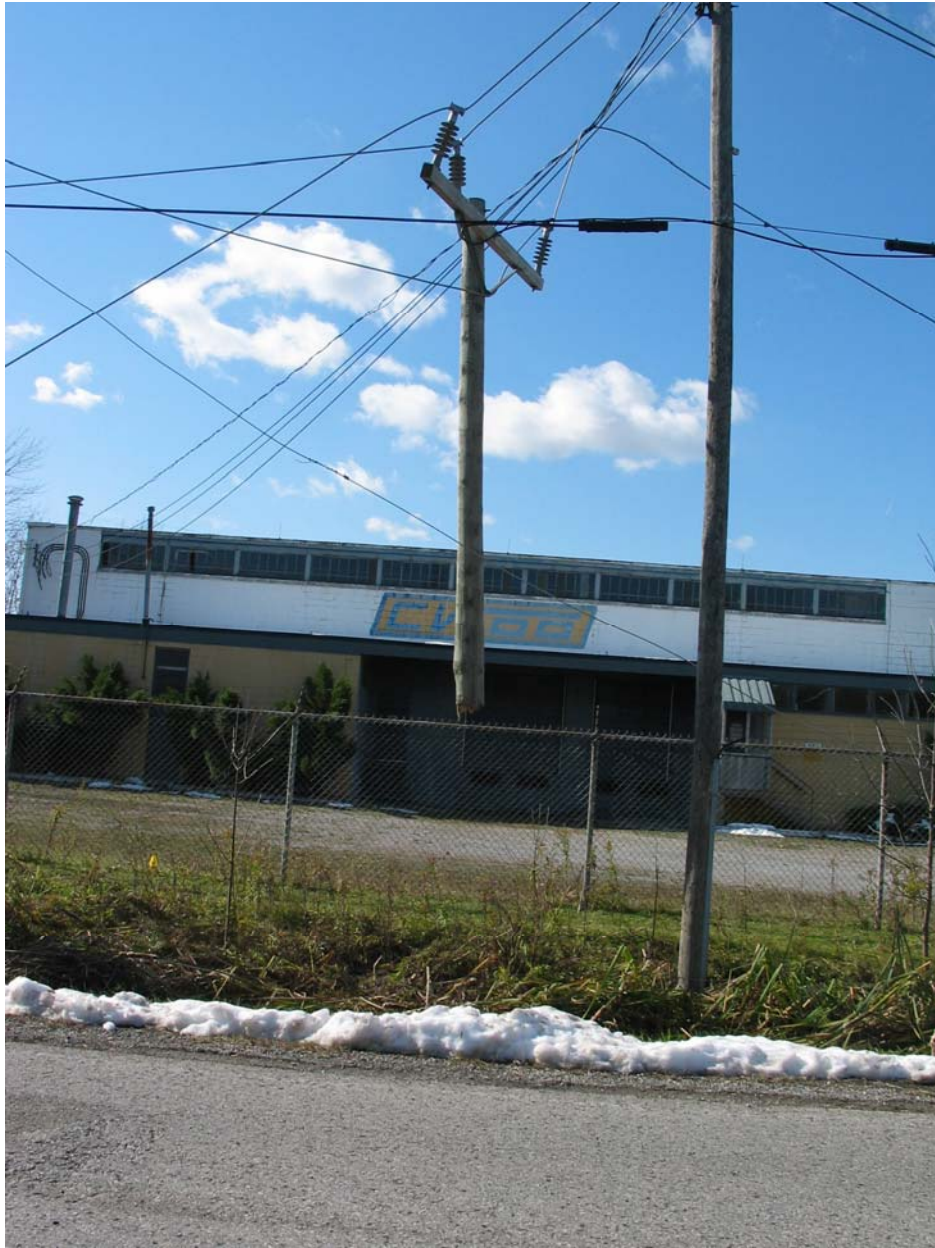
Poles shear from loading of snow, wind and trees.
