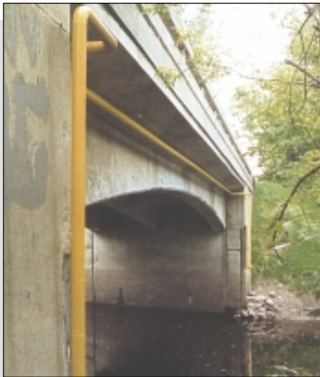
Attaching gas line on a bridge.
