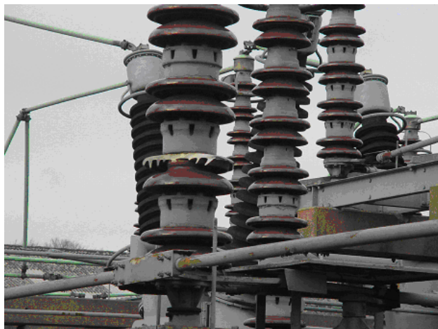
Figure 11: Cracked Insulator Porcelain – 3 rd from Bottom
